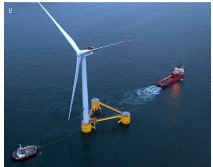
Figure 2.5 A: Hywind Scotland spar floating wind turbine; B: WindFloat Atlantic semi-submersible floating wind turbine.
