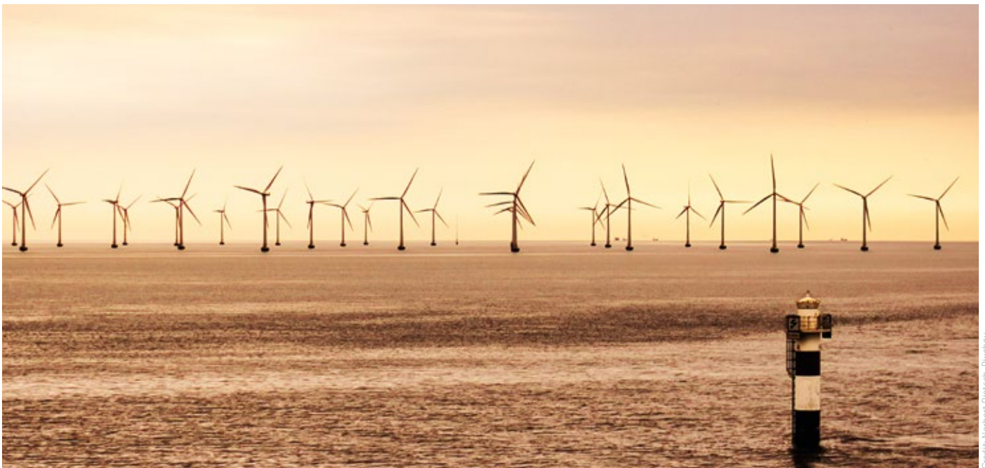
Wind turbines at sea.
