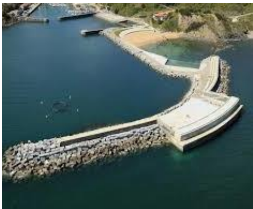
Figure 2-1 Mutriku wave energy plant [11].
